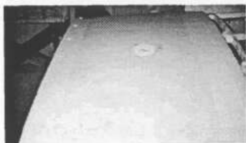
Completed flush-mount filler cap for header tank. Deck secured to tank with machine screws and nutsert fittings. Preplan instrument panel installation during deck fitting process.
