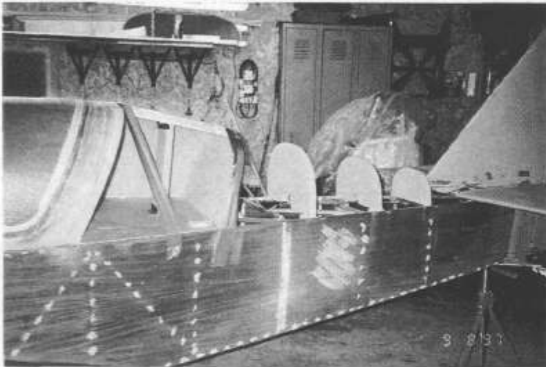
One-inch thick foam formers support aft turtledeck structure.
